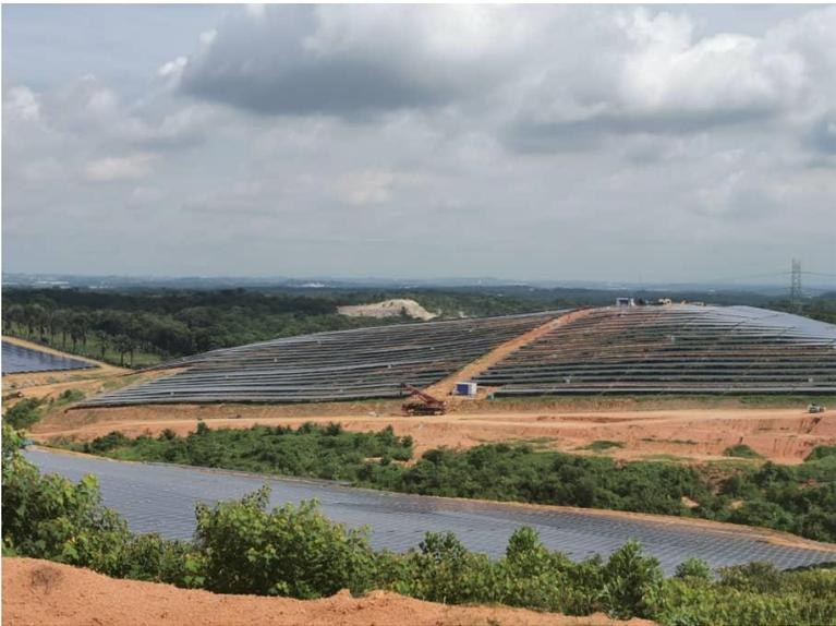
UiTM Solar Park II's fixed tilt ground-mounted solar panel polycrystalline silicon PV modules retains natural topography of undulating site terrain. Photo credit: KY Chia
